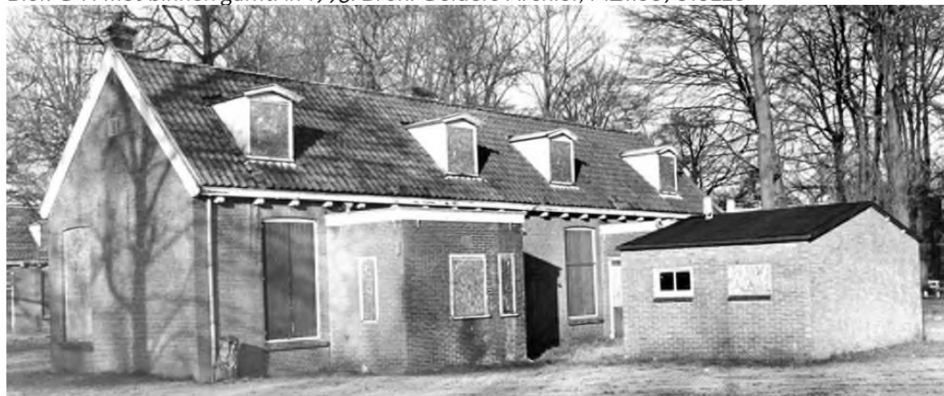
Blok E-F in 1993. Bron: Gelders Archief, MZ11607010233
