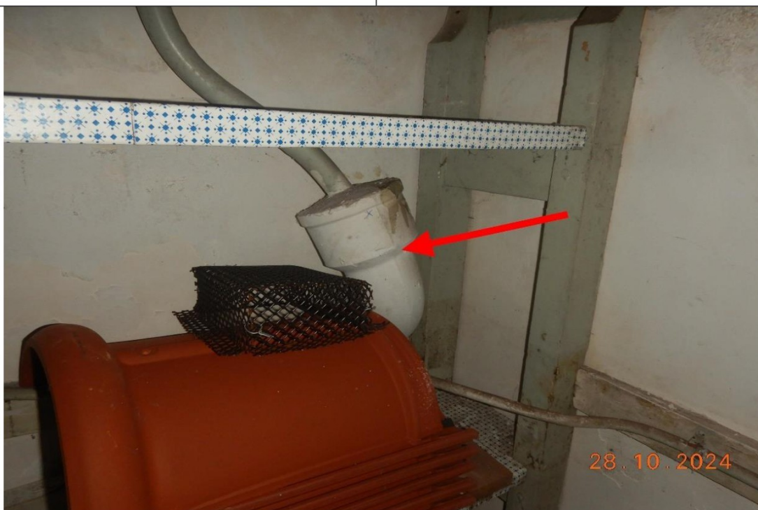
Foto 69 | Riolering in hoek
