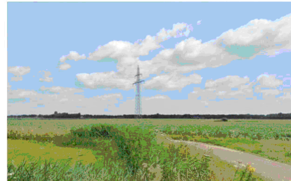
1 st electricity pylon
